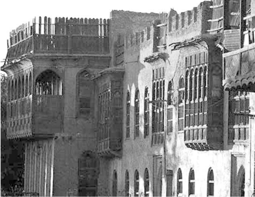
Shanashil (bay windows) of old houses in Bara, Iraq.
